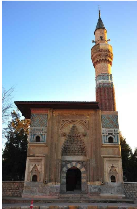
Figure 2. The main gate of the Sahip Ata Complex and the sebils located on both sides (URL 1)
