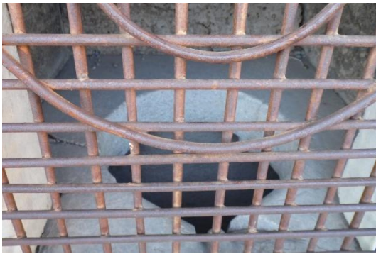
Upper Part of the Chamber
